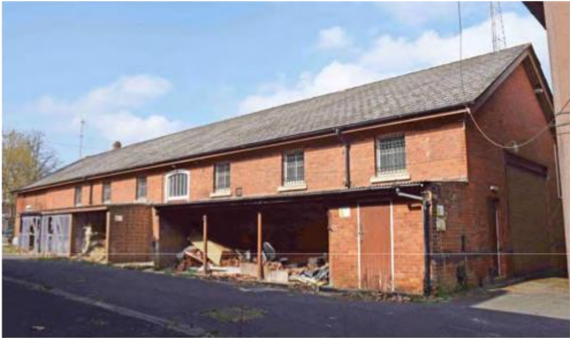
View from the north-east of Building 14E
