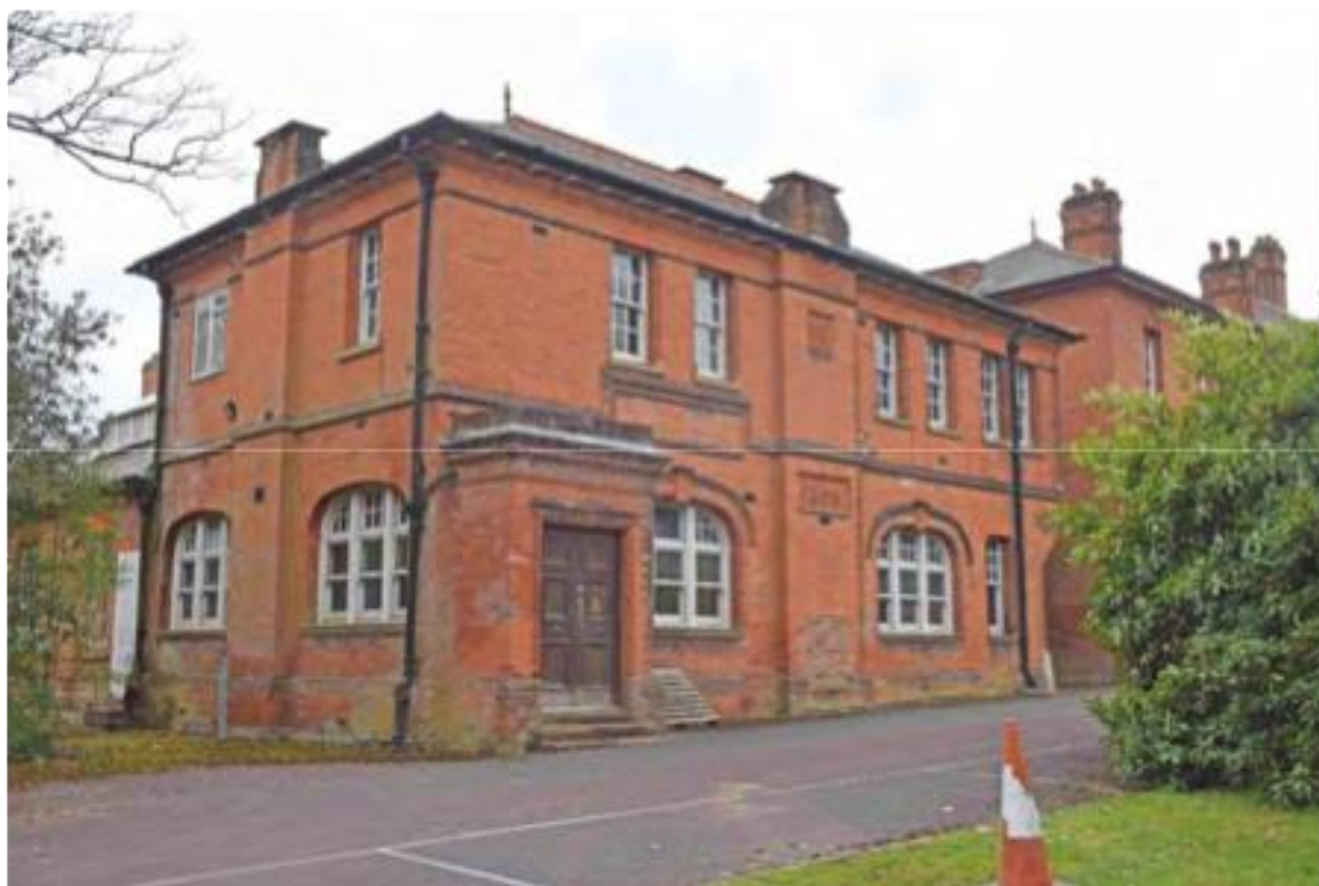
View from the north-west of the Post Office
